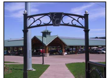
Farmers Market Pavilion completed
